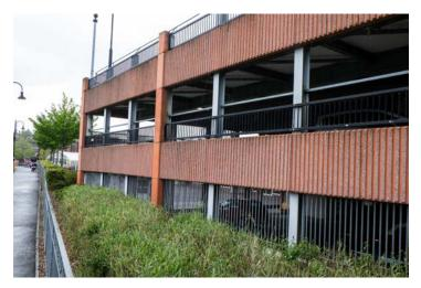
Note the railings on the ground floor. Similar railings should be put along this edge of the second floor to prevent access.
